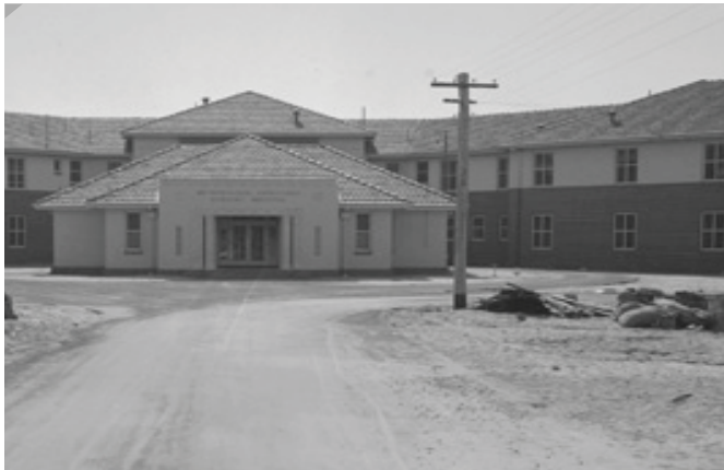
Archival Image 3 The new Infectious Diseases Hospital administration and ward buildings nearing completion in 1938 (Source: SLWA online image call no.09480PD)
