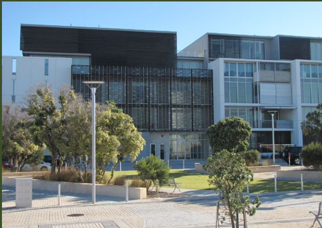
Building with a variety of facade depths and articulated volumes with consideration for different levels of shading, privacy screening, and acoustic separation
