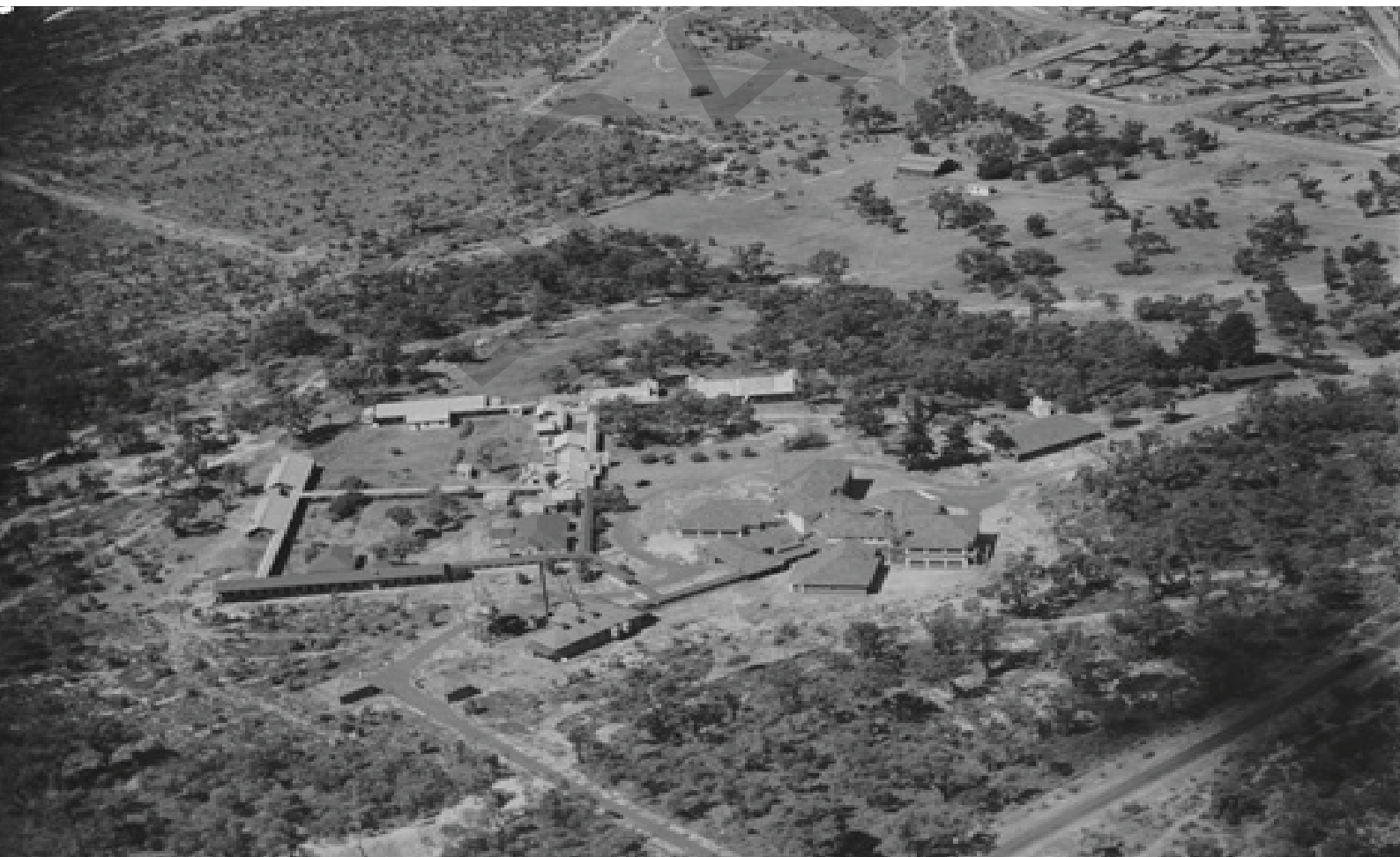
Archival Image 1: ca.1938 aerial image of the SPRH site following construction of the new Infectious Diseases Hospital administration and ward buildings (Source: SLWA online image call no.031661PD)
