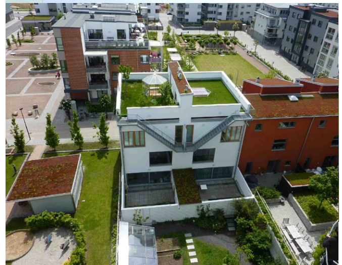
An example of a well considered roof elevation from adjacent taller buildings
