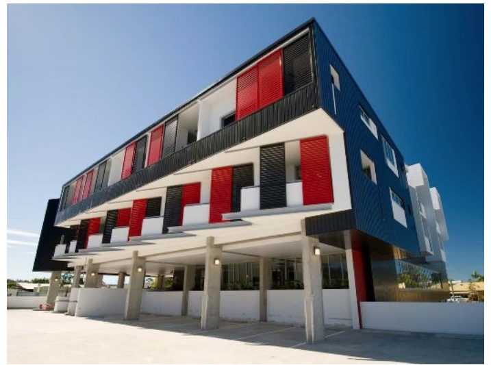
Undercroft parking to the rear of a site not visible from the street.
