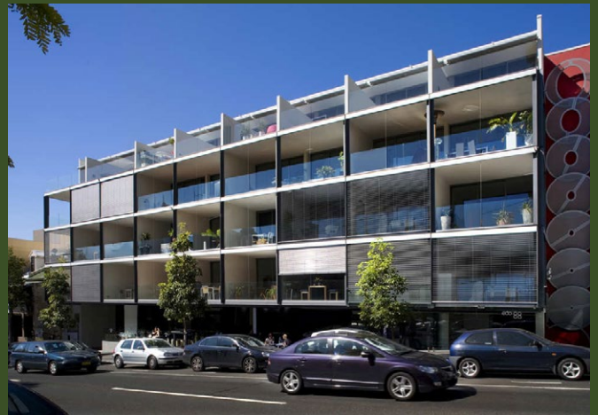
Examples of shading devices to windows and balconies promoting building articulation and material variety
