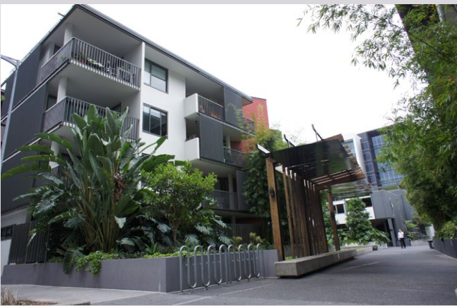
Corner residential ground floor apartment or terrace
