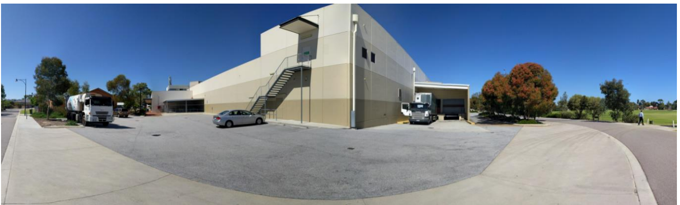
Figure 15 View of minor car park (left) and the loading dock area (right) .
