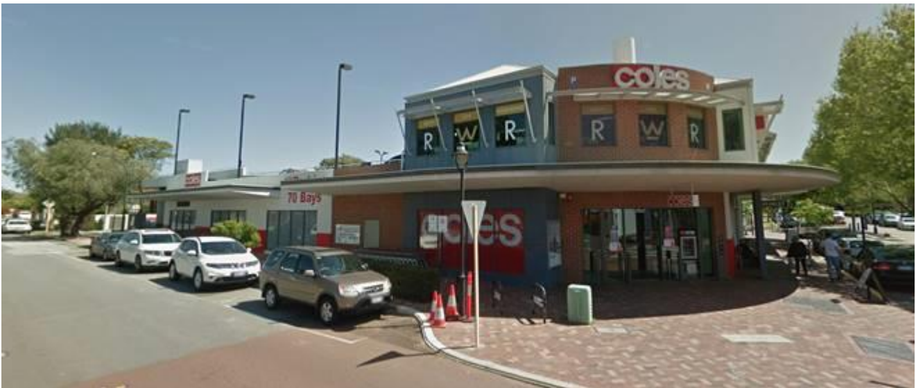
Figure 17 Angelo Street, South Perth. Concealed deck parking (left).
