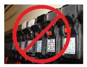
These devices only cut the flow of electricity when a high level of electrical leakage is detected.
