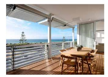
**Photo G2.2a** Adjustable louvres are an effective way to control sun, glare, privacy and ventilation through the day and year (PC)
