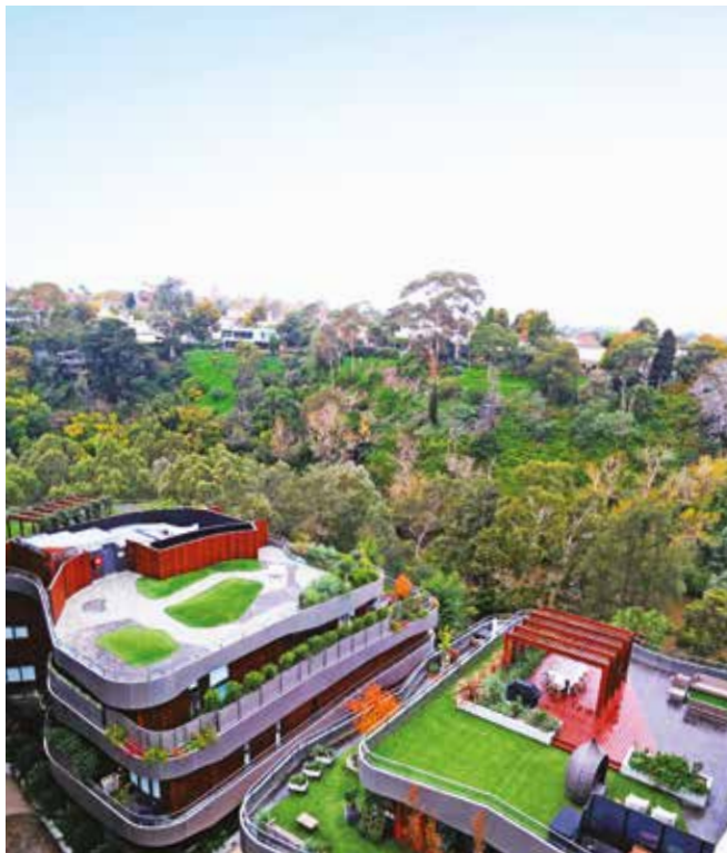
Photo 4.11a Open space, landscaping and other amenity provisions are maximised on these roof and balcony spaces.
