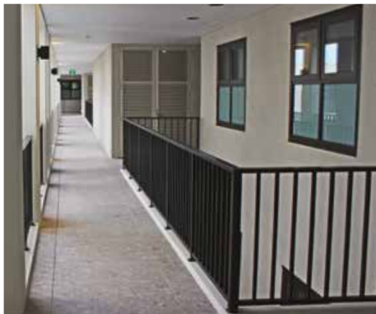
Photo 4.6a Storage cabinets are integrated at the entrances of the dwelling units in this development, making them convenient to use, easily accessible and more secured.
