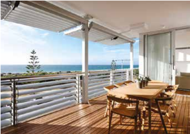
Photo 4.1c Louvred balustrades and operable awnings allow residents to adapt the balcony for light or shade throughout the day, as well as controlling shelter and privacy. (PC)
