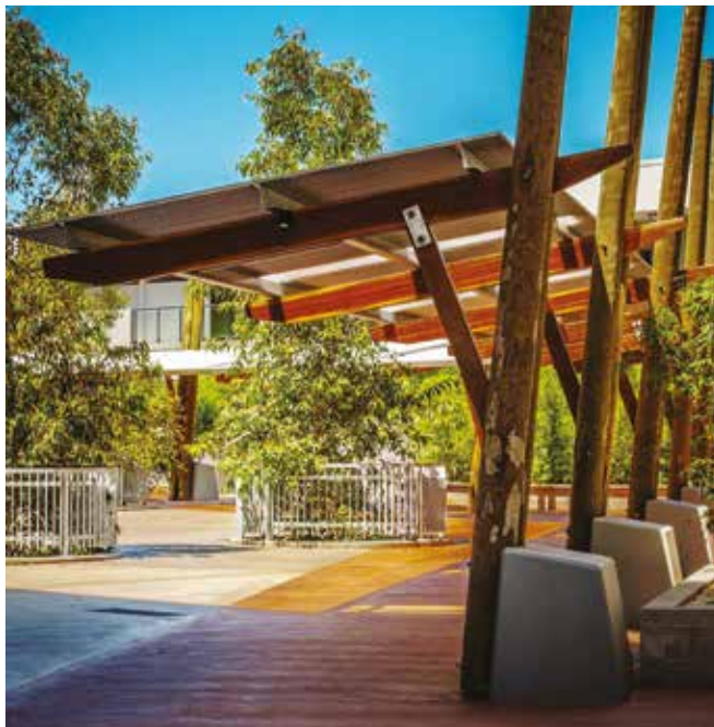
Photo 4.12a Well considered landscape design can add significant amenity to communal areas. (PC)
