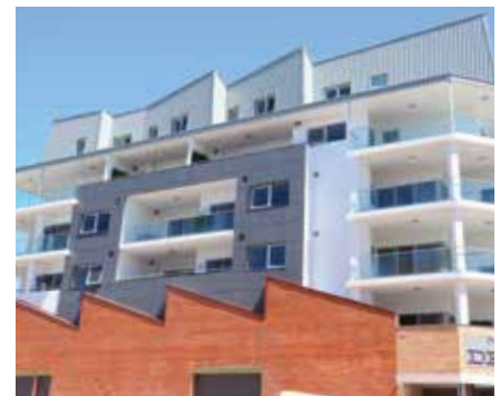
Photo 4.11c The roof line of this development mimics the original building's roof structure.
