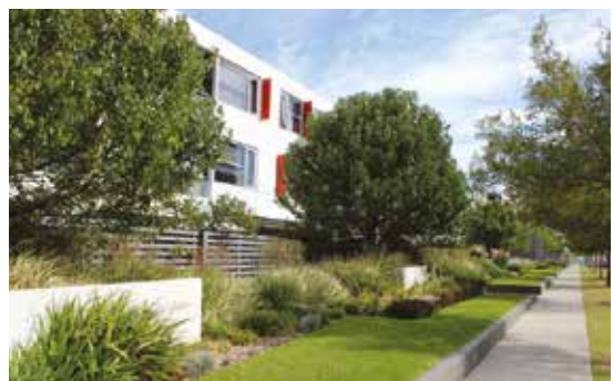
Photo 3.6c The landscaping in front of these buildings contribute to a positive streetscape character, with building frontages and entries onto the street. The multiple entrances also help to activate the street edge, while providing passive surveillance over the public street.
