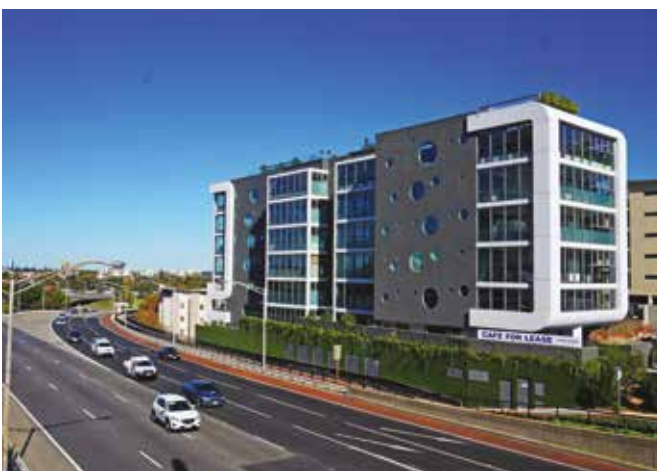
Photo 4.7b Development next to a freeway needs sufficient noise abatement measures such as those listed in DG 4.7.3. (See also Photo 4.7c, showing some of the noise reduction features in the same building).
