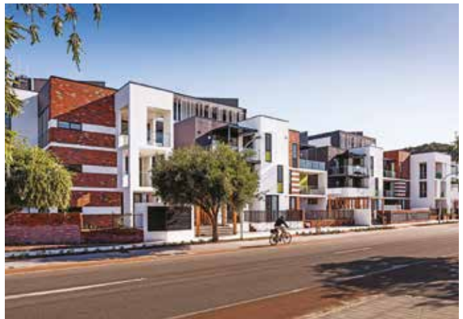
Photo 3.6g An eye level/street view of the same development in Photo 3.6h below, showing how the building interacts with the street defining the streetscape for the area. (PC)
