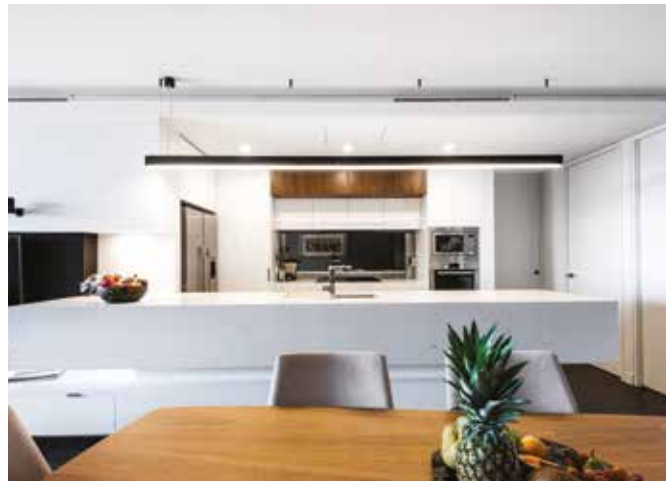
Photo 4.3b Bulkheads concealing mechanical services can also serve to delineate spaces in an open plan layout. (PC)
