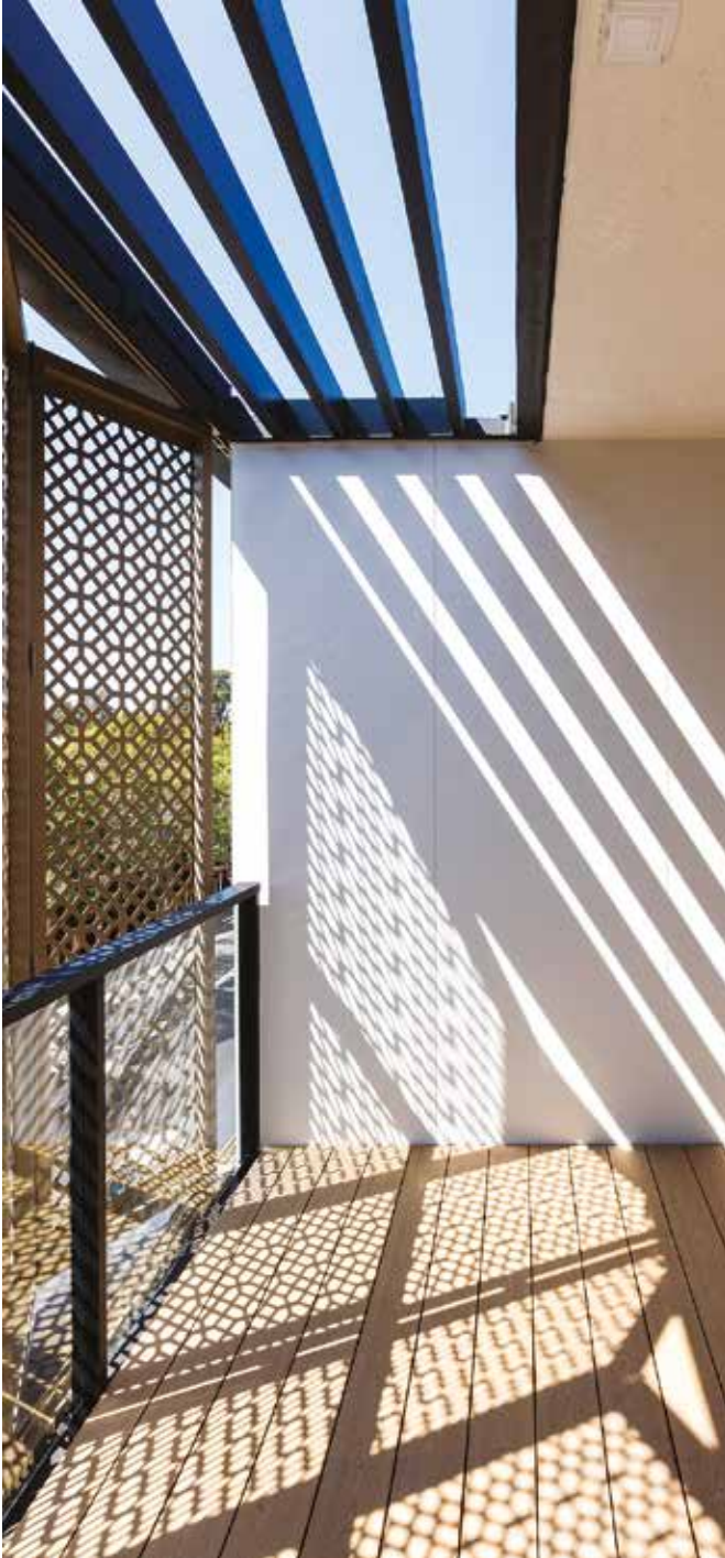
Photo 4.2a Sun screen and pergola structure provide shade and at the same time allow for natural ventilation. (PC)
