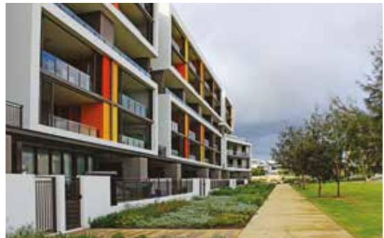
Photo 3.6a The upper level balconies of this development overlook public open space providing the residents with an attractive outlook while providing passive surveillance of the public domain.
