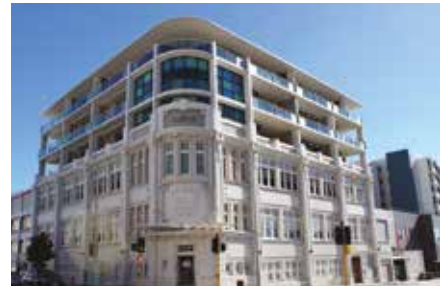
Photo 4.13a Additional levels of apartments reinforce characteristics of the existing heritage building while remaining modern and distinct.
