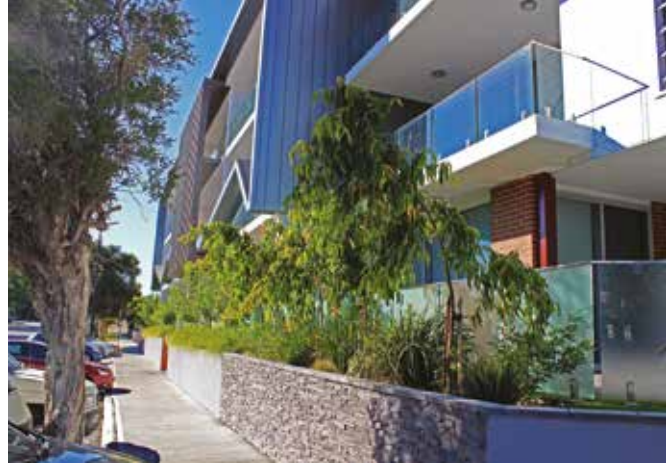
Photo 3.6e The raised planter and landscaping enhance the privacy of these ground floor apartments, improve the public domain interface and at the same time contribute to the greening of the streetscape.
