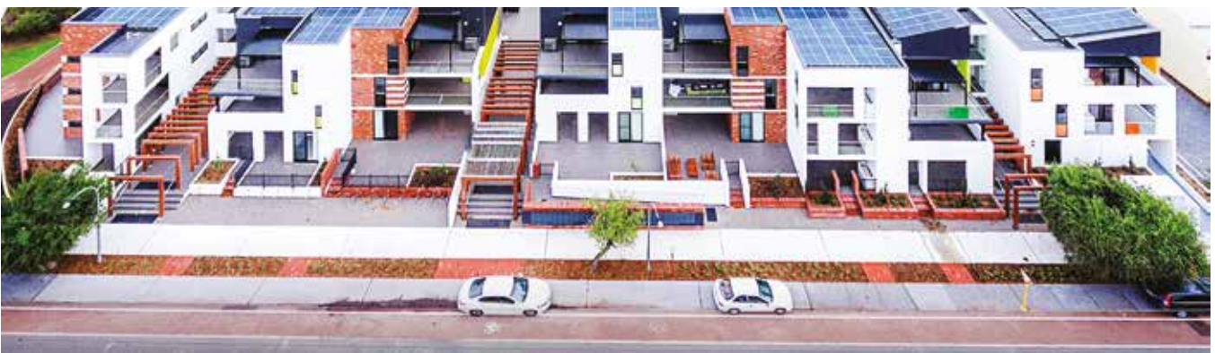
Photo 3.6h Some good public interface elements are demonstrated here: the three street entry points are clearly legible, one of them has universal access; change in level between footpath and front courtyards for privacy allowing for largely permeable fencing; upper level balconies and windows overlook the street and public domain areas ensure public surveillance; mix of textures and materials provide pedestrian interest; mail boxes and bike racks are well integrated along front fences; landscaping provision is generous and enhances the layout design. (PC)
