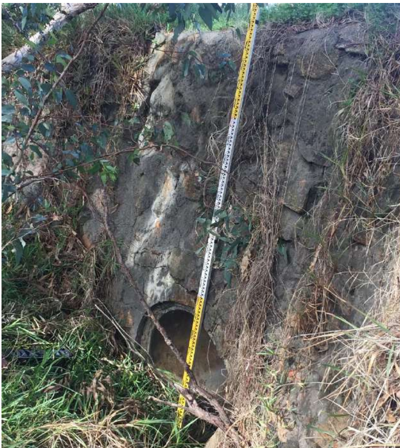
PLATE 8: 900 mm dia pipe under Muriel St. Invert of pipe is several metres below road level.
