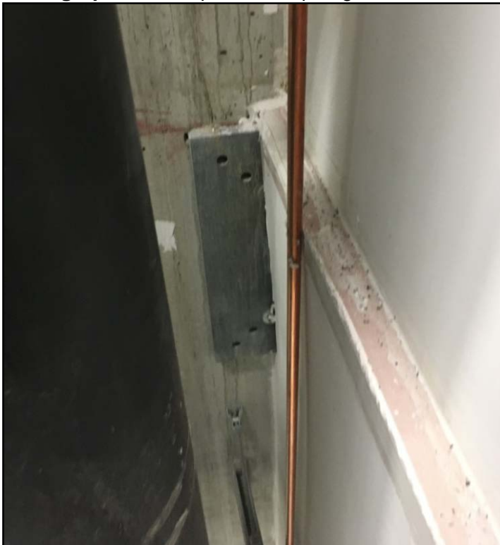
Photograph 2: Example of a strip of glued-on fire rated plasterboard
