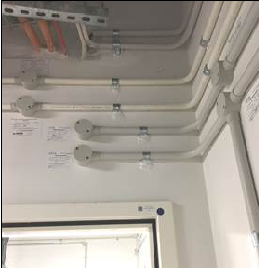
Photograph 4: Example of hollow wall non-fire rated fixings in a fire rated wall
