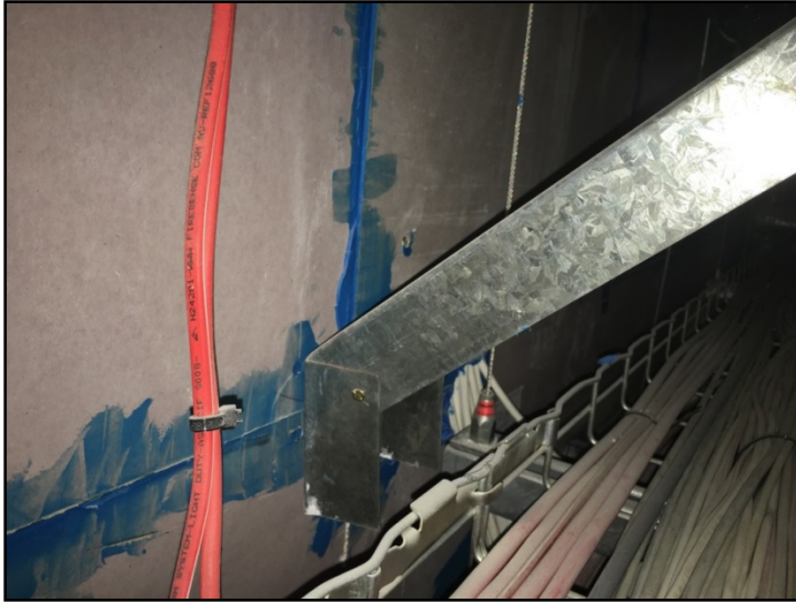
Photograph 1: Wall brace fitted to a plasterboard wall
