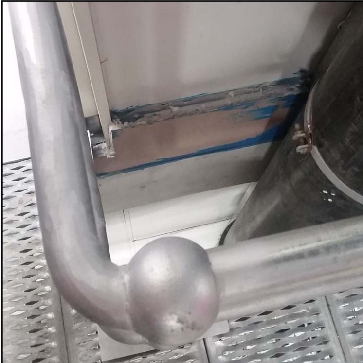
Photograph 3: Example of a strip of glued-on fire rated plasterboard
