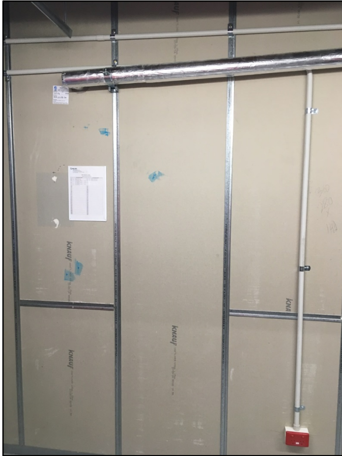
Photograph 13: Saddle clamp fixings to inside face of Knauf shaft wall
