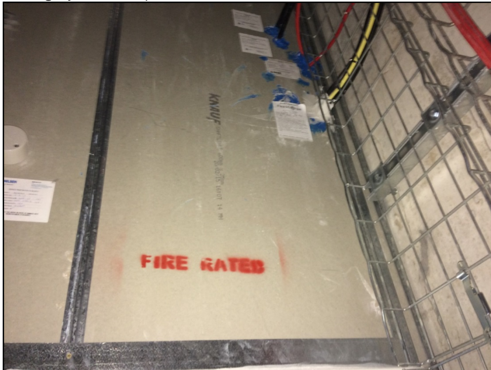
Photograph 8: Example of labels and fire stencils
