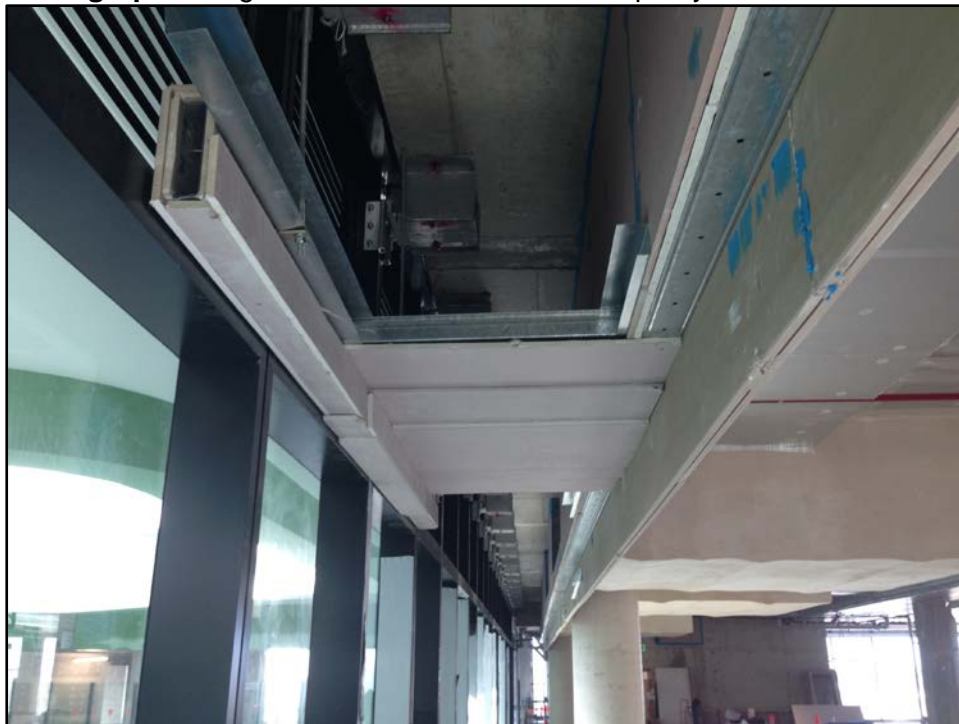
Photograph 9: High level louvre air intakes and partly constructed air duct
