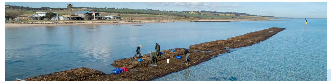
A shellfish reef breakwater for erosion control being seeded with native mussels at Portarlington, Port Phillip Bay, VIC. Photo: Reg Ryan
