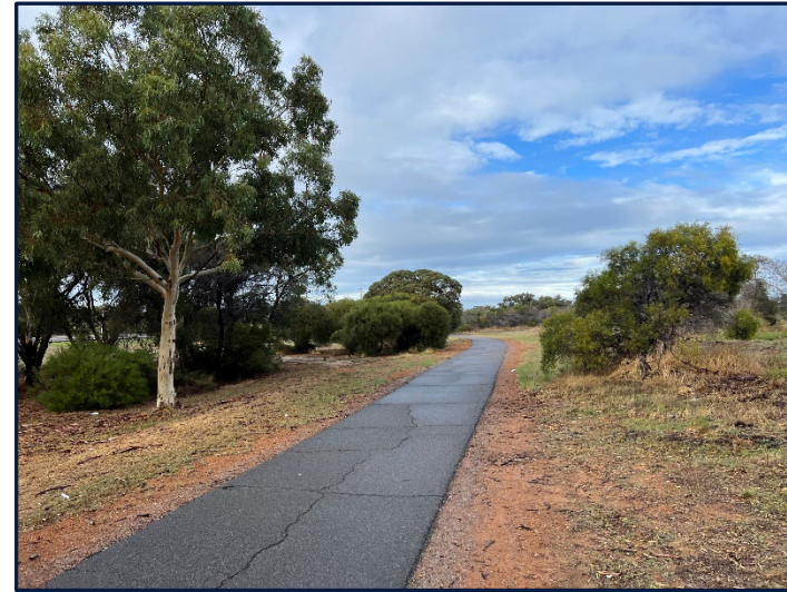
Figure 5 Existing dual use path on eastern boundary
