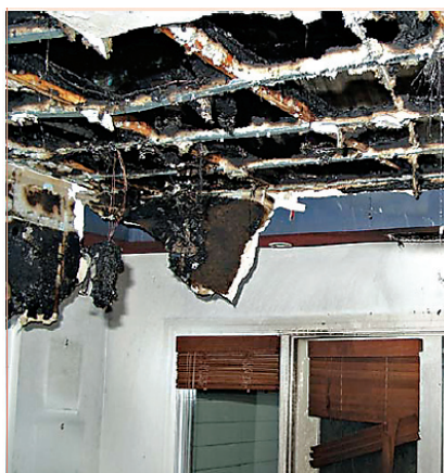
Damage caused by a ceiling fire attributed to downlights.
