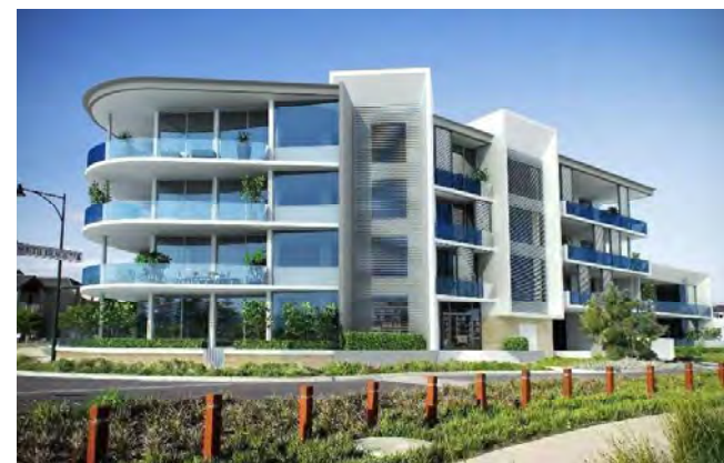
Photograph 33. A combination of open, solid and adjustable elements facilitate optimised airflow
