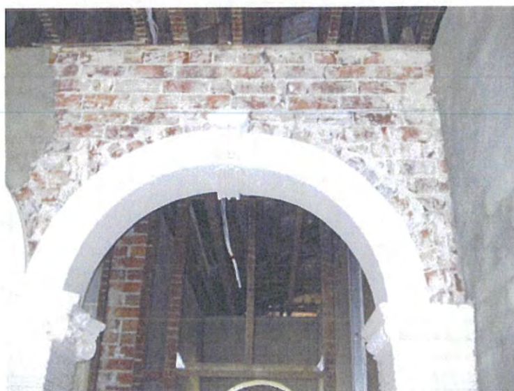
Ornamental Plasterwork - Extent of cracking in internal walls upper floor.
