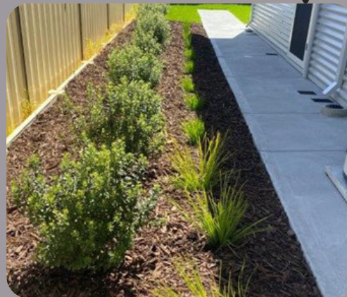
Figure 125. 1m concrete apron installed to perimeter of dwelling and graded toward garden beds. Low maintenance species planted at required 2 plants/m 2 .
