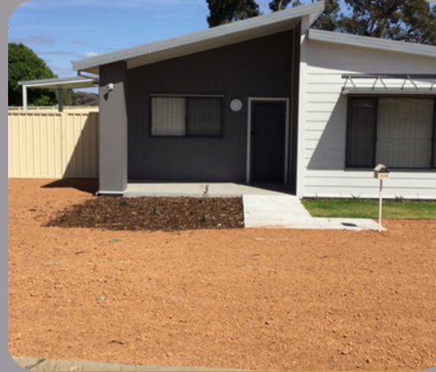
Figure 108. An excessive use of gravel treatment and turf located directly against the dwelling.
