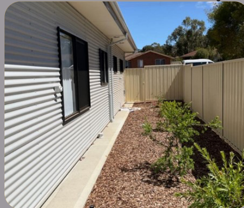
Figure 117. Concrete apron installed. Small shrubs installed to minimise conflict with fence or dwelling.
