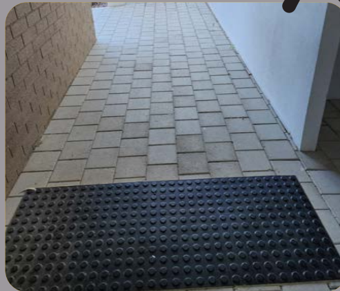
Figure 90. Stick on TGSI's are not sufficiently robust. TGSI's only required where ramps or stairs are needed.
