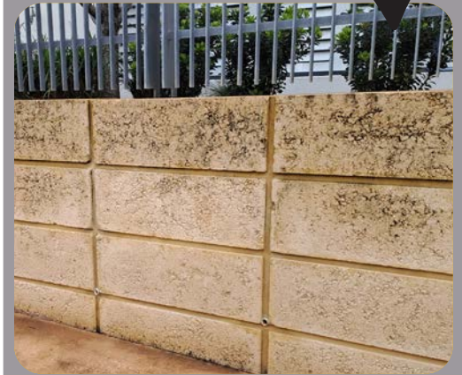
Figure 73. Limestone block with integrated boundary fencing is a preferred construction method.
