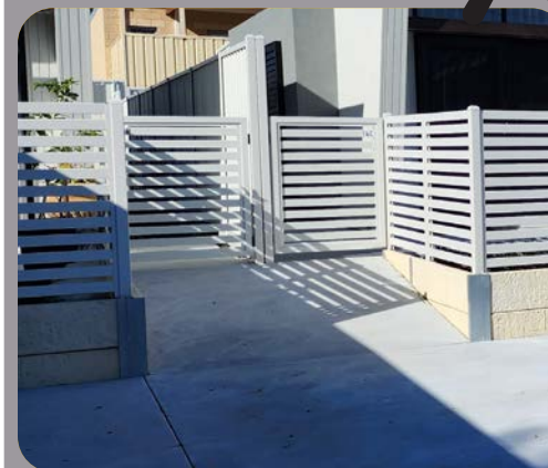
Figure 88. Primary entries to dwellings are steep with non-conforming ramps, no handrails, kickguards or TGSIs
