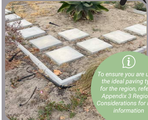
Figure 22. Height of gap between pavers is a trip hazard. Space needs to be filled in with material to maintain flush edge.
