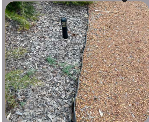
Figure 68. Thin plastic or steel edging is not robust and is not to be used.
