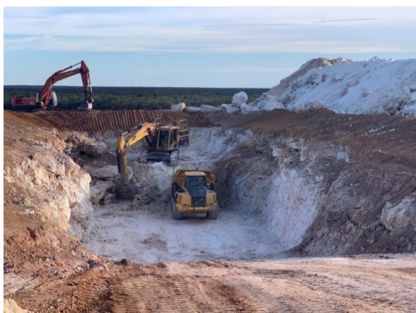
Excavation of the 2020NRT01 Disposal Trench
