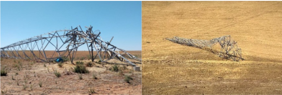
Figure 8: Transmission tower damage (from DEMIRS 2024).
