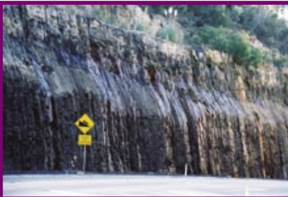
Fig 9. A raised ground water level may be evident in road cuttings after periods of abundant rainfall
