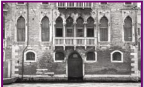
Fig 35. Capillary rise of sea water in an old building in Venice (Reference 22)
