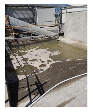
No water used in concrete batching or cement product manufacturing can be discharged from the premises until it has been through a silt trap or contained in a settling pond for long enough to allow all particulate matter to settle out. Additionally, if the water is likely to contain hydrocarbons it also needs to go through an oil interceptor.
