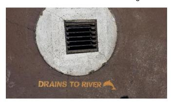
harmful materials. This includes stormwater that may have picked up contaminates from industrial areas such as hardstands. The runoff which enters the stormwater drain is carried in underground pipes or open ditches and discharged untreated into local streams, rivers and other wetlands and surface water bodies.
