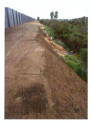
Plate 17: Acoustic wall installed in the northern portion of Lot 9001 Mortimer Road, adjacent to the Kwinana Freeway showing firebreak and interface with vegetation.
