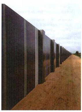
Plate 18 Acoustic wall likely to be installed adjacent to north-west boundary of the site, approximately 3m high with 3m-wide firebreak
