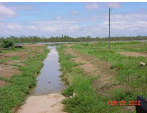
Figure 10 - drainage channel between Lts 34 & 36 mitigating high water levels in 2002
