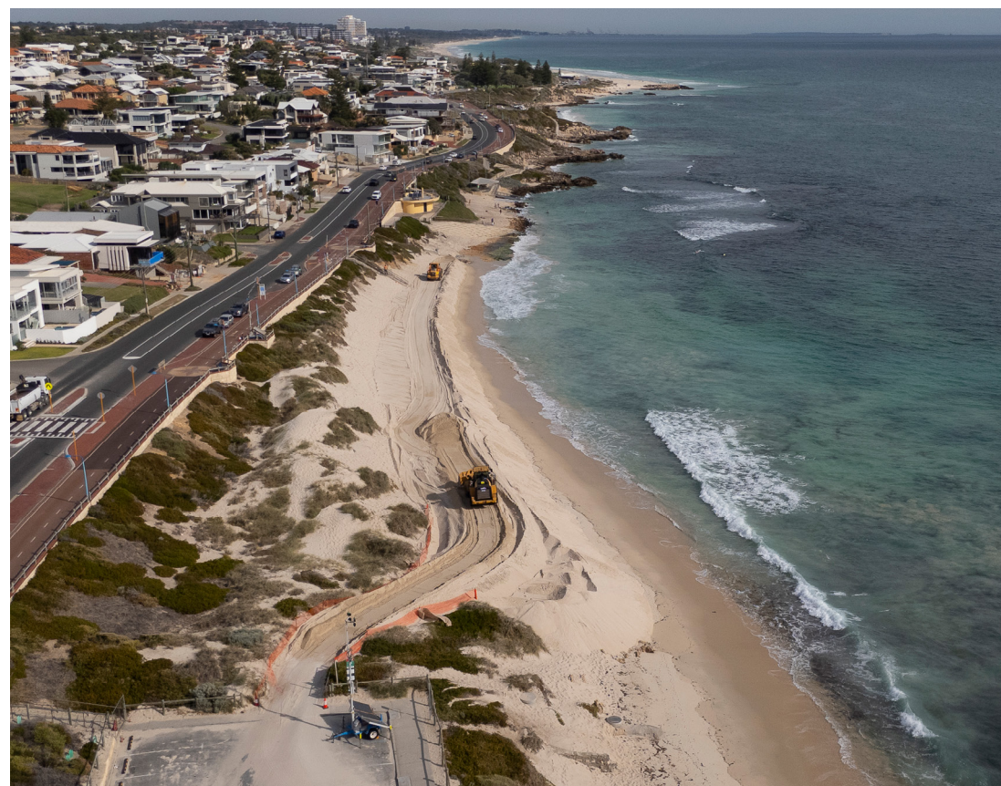
Sand nourishment project at Mettams Pool (image sourced from City of Stirling)
