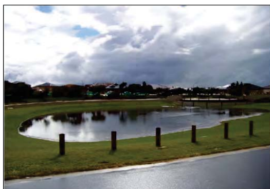
(Top left) Dry basin landscaped swale within multiple use function restricted use public open space (Top right) Landscaped dry basin in POS after storm event
