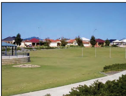
(Top left) Dry basin landscaped swale within multiple use function restricted use public open space (Top right) Landscaped dry basin in POS after storm event
