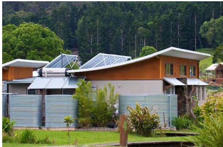
Figure 6: Example of energy efficient housing design utilising photovoltaic panels, passive solar design and on-site water supplies.
