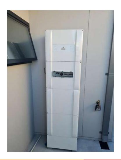
**Inadequate clearance around BESS**
