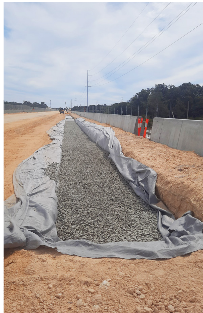
Rail ballast reused as drainage in road construction
