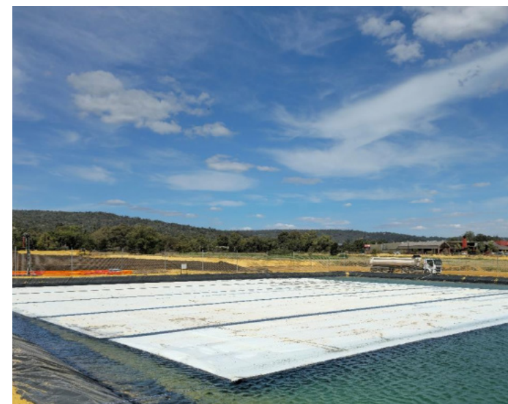
Dam covers made 30 per cent recycled material, later reused in rail extension project
