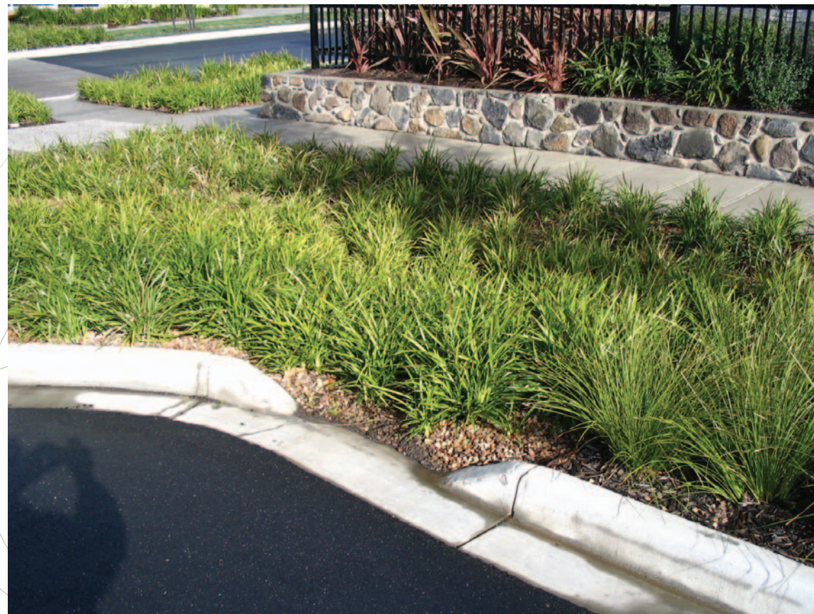
End of street bioretention unit
