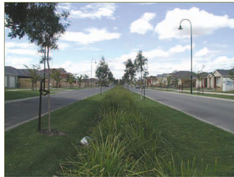
Linear bioretention swale in multiple use corridor
