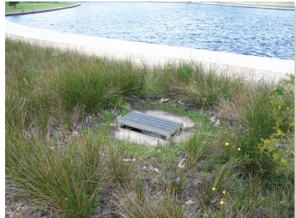
Bubble up pit in Bioretention Basin
