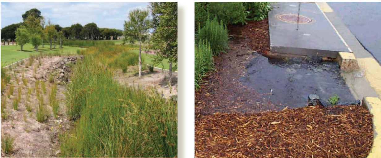
Swale Drain Bioretention Unit
