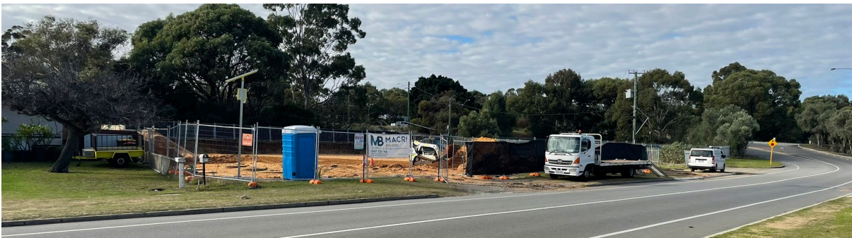
Photograph 3: Looking south east towards R60 residential development site.
