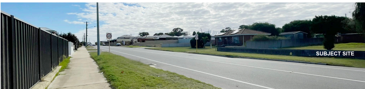
Photograph 4: Looking north west along Rockingham Road towards R40 development sites under construction nearby the subject site.
