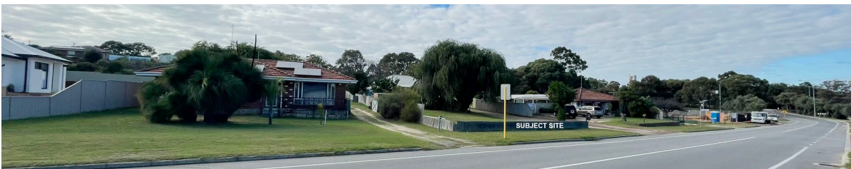
Photograph 2: Standing on the western side of Rockingham Road, looking south east towards the subject site and subdivision works for the R60 residential development underway nearby the site.
