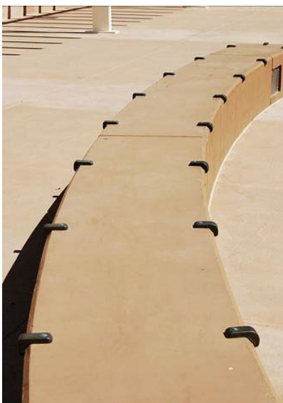
Figure 2: Anti-skateboard fixings must be vandal resistant.
