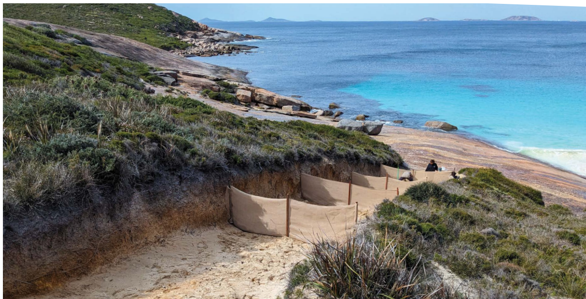
Dune forming fence work, Tjaltjraak Boodja Park Stage 3 Coastal restoration.
