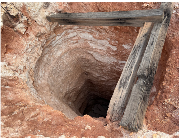
Cue phase 1 stage 1 geotechnical assessment in progress. Left: Open abandoned mine shaft with erosion evident around original timbers. Right: Down-hole LiDAR scanning of abandoned mine feature with eroding collar.
