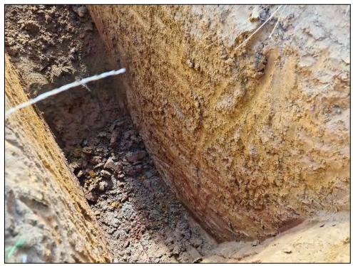
Figure 14: Test Pit 7 Soil Profile
