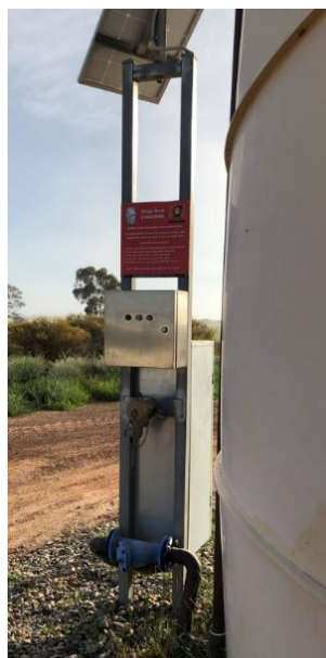
Swipe card standpipe system
