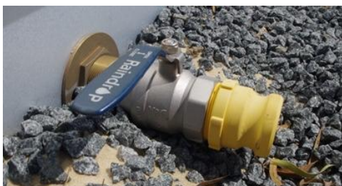
Tank standard camlock fitting
