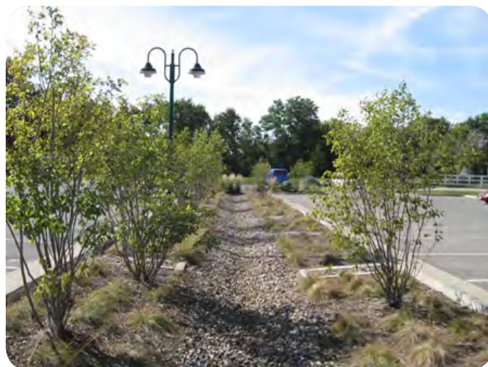
Examples of drainage infrastructure recommended by the local water management strategy; swale within open space (top); roadside swale (centre and bottom).
