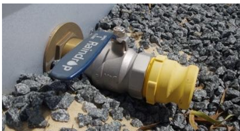
Tank standard camlock fitting
