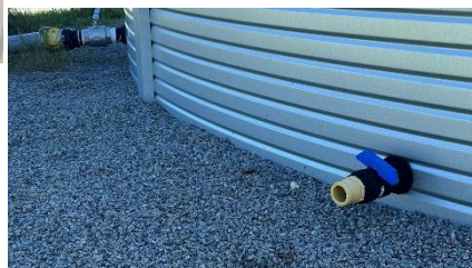
Left: bore and pump Right: 100mm suction outlet Below: 50mm outlet
