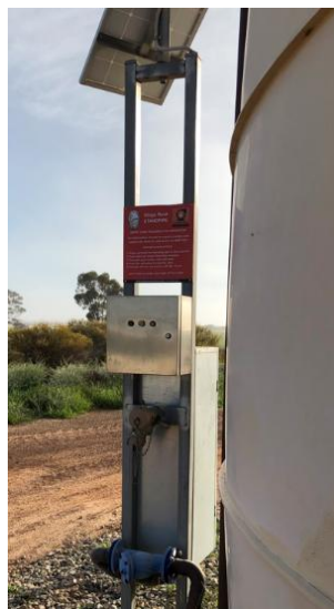
Swipe card standpipe system
