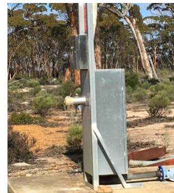
Coupling on standpipe
