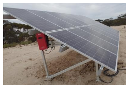
Solar pump and panels
