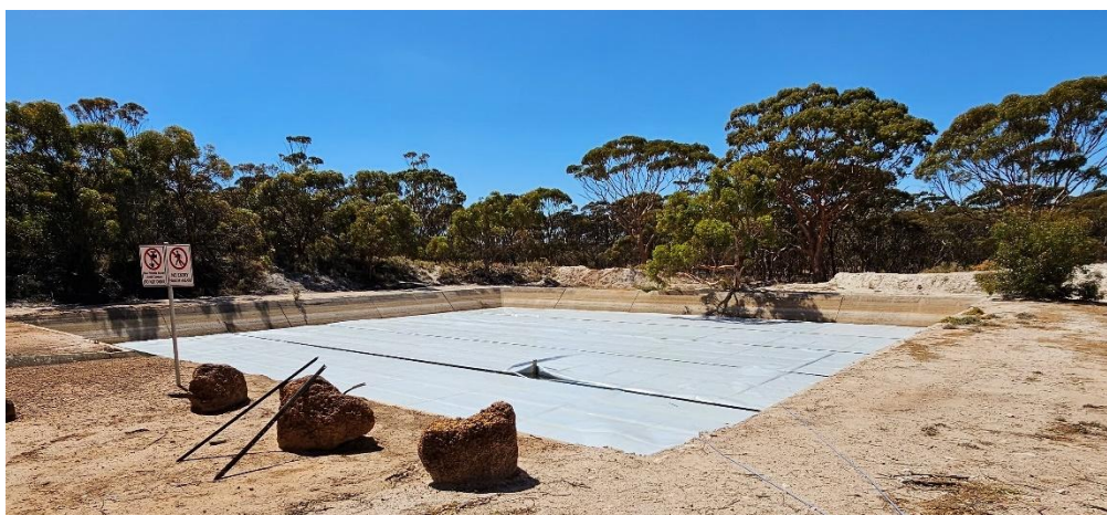
Lake Grace north dam with daisy covers installed
