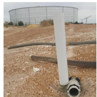
Coupling outlet near tank
