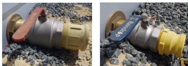
Coupling outlets on tanks
