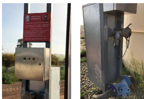
Standpipe signage and coupling
