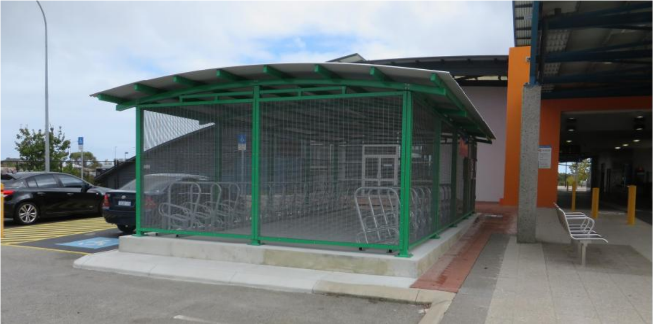
Figure 2-11: Bike Parking Shelter at Wellard Station
