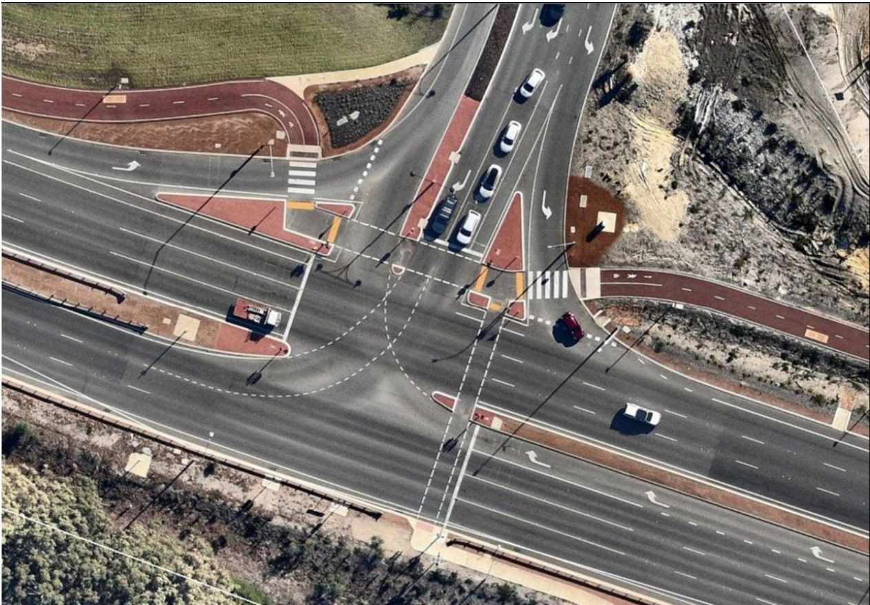
Figure 3-3: Typical intersection St Albans Road / Mundijong Road (Ghostgum Ave, Armadale Rd)
