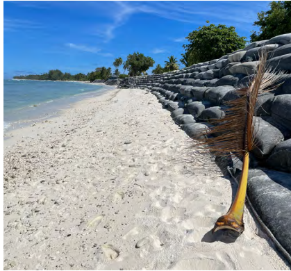
MU1: West Island Settlement - GSC sandbag seawall
