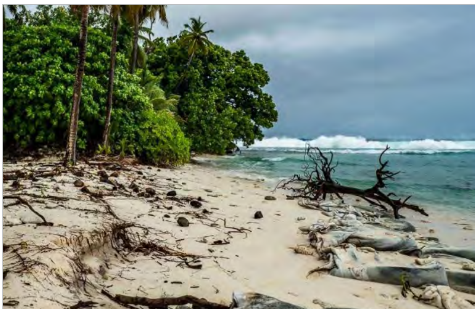
Figure 14: Trannies Beach erosion and failure of seawall following July 2018 event (RHDHV, 2021a – source: Karen Willshaw)
