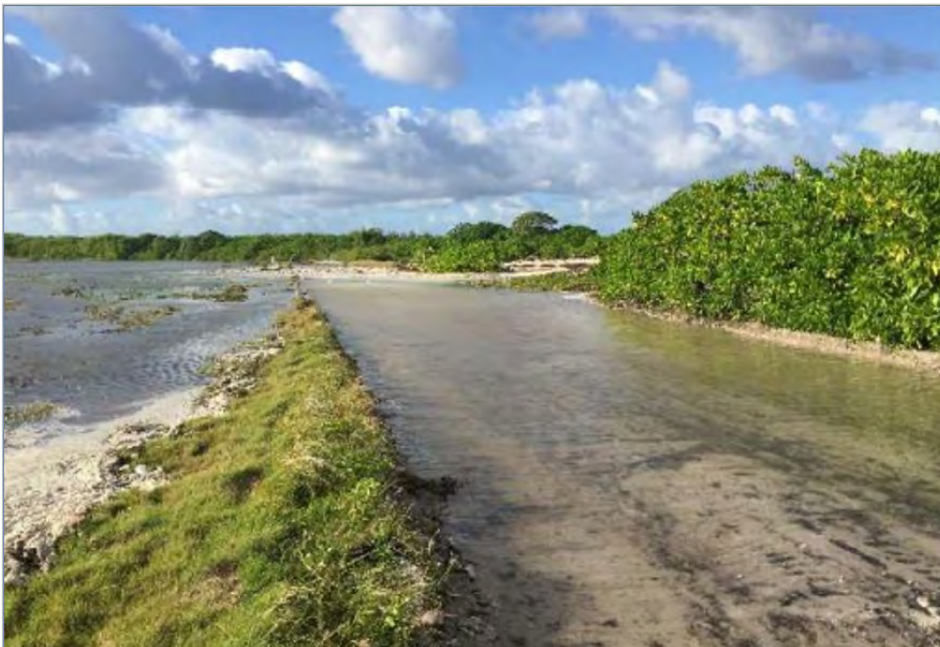
Figure 16: Airforce Road flooding during July 2018 storm event (RHDHV, 2021a – source: David McKinney)
