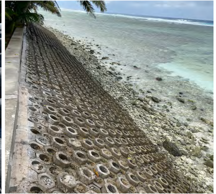
MU1: West Island Settlement - Seabee seawall
