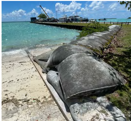
MU 7: Home Island Settlement - Ferry wharf and infrastructure
