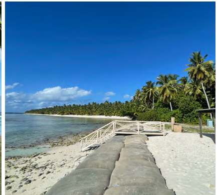
MU 2: West Island Ocean Beaches - GSC sandbag seawall Trannies Beach
