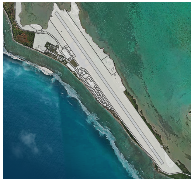
Figure 57: West Island whole of settlement
