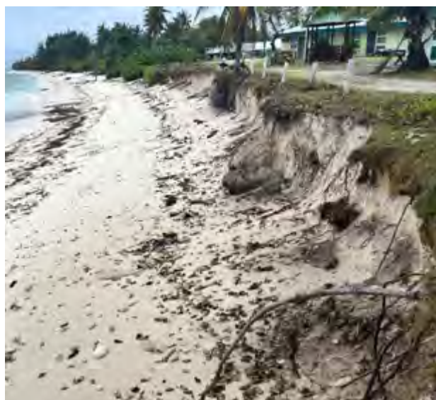
Figure 40: Chronic erosion of ocean facing foreshore fronting settlement in West Island
