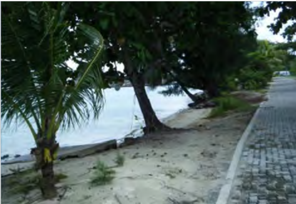
Figure 12: Jalan Pantai on Home Island prior to seawall construction (2) indicating the low elevation of the road and narrow foreshore, 29 May 2009 (DoT, 2010)
