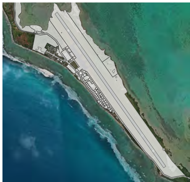
Figure 57: West Island whole of settlement
