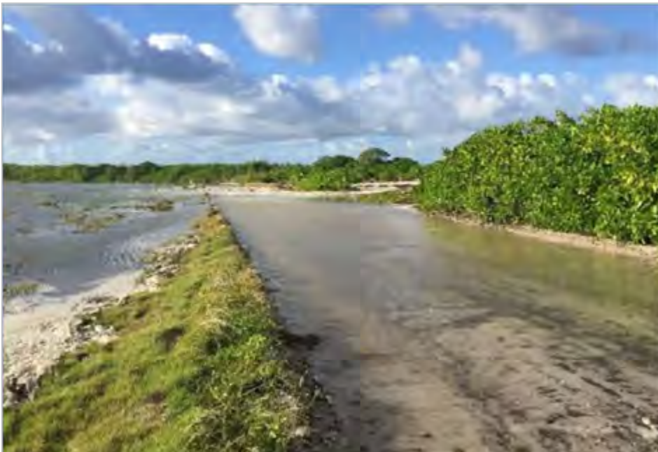
Figure 16: Airforce Road flooding during July 2018 storm event (RHDHV, 2021a – source: David McKinney)
