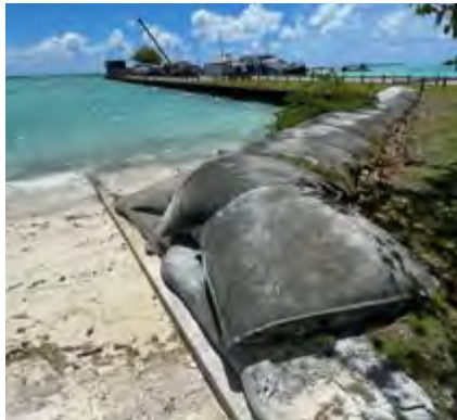
MU 7: Home Island Settlement - Ferry wharf and infrastructure
