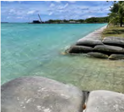
MU 7: Home Island Settlement - Jalan Pantai seawall
