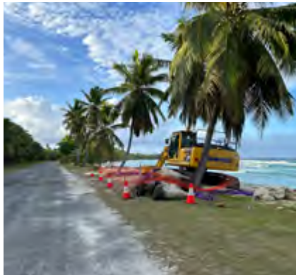
MU 2: West Island Ocean Beaches - GSC sandbag seawall under repair
