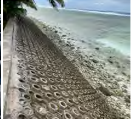
MU1: West Island Settlement - Seabee seawall
