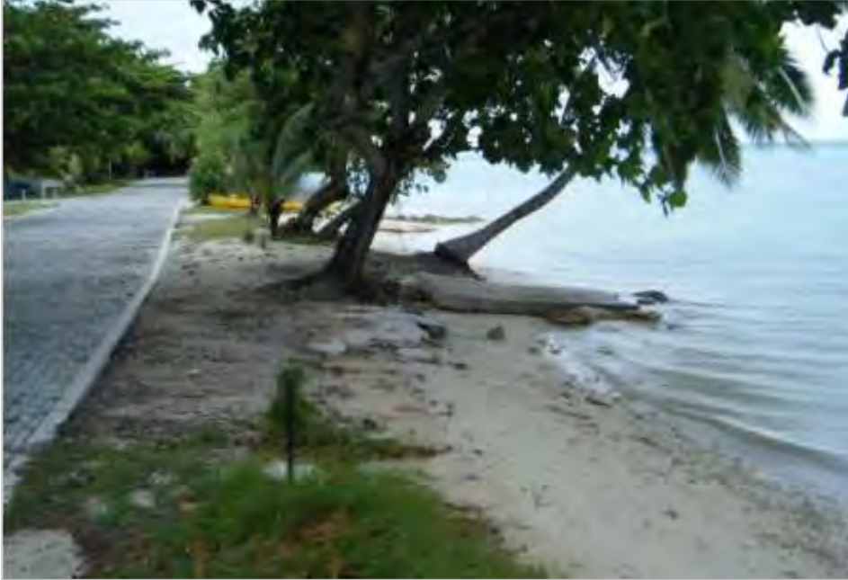
Figure 11: Jalan Pantai on Home Island prior to seawall construction (1) indicating the low elevation of the road and narrow foreshore, 29 May 2009 (DoT, 2010)
