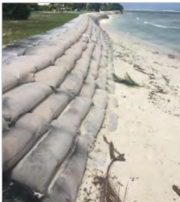
Figure 21: Photo of William Keeling GSC seawall as an example of a typical GSC seawall (RHDHV 2021b)
