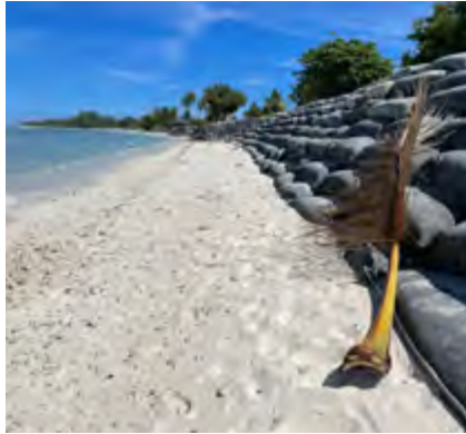
MU1: West Island Settlement - GSC sandbag seawall
