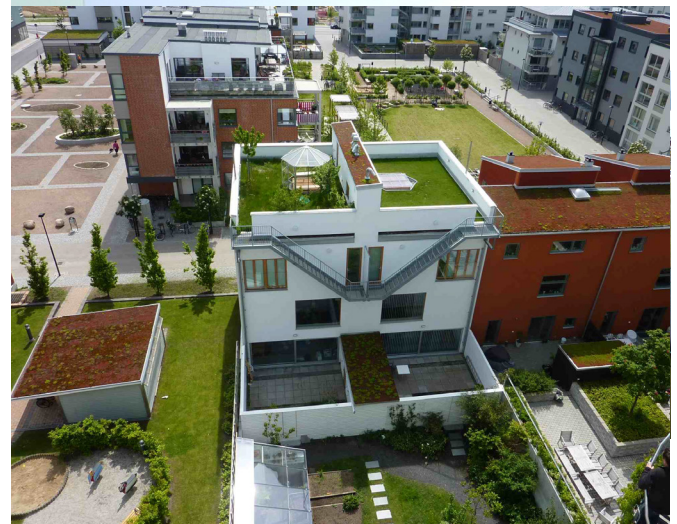
An example of a well considered roof elevation from adjacent taller buildings
