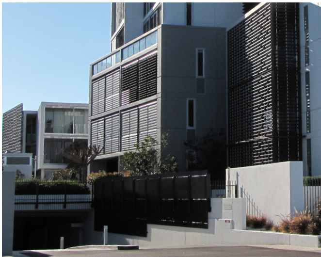
Discrete vehicle entries designed to minimise view from the street
