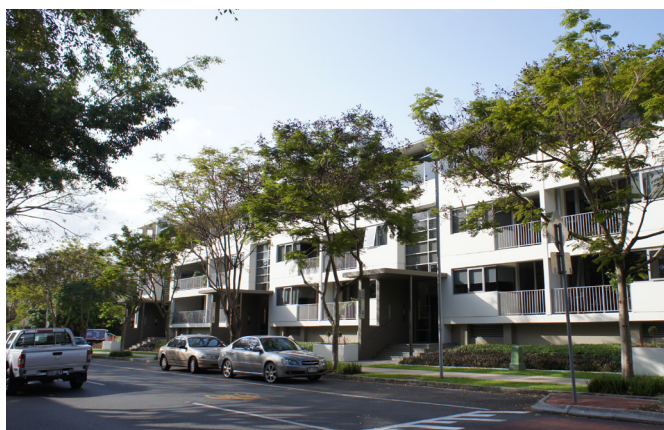
A podium level between three and four storeys creates a well proportioned human scale streetscape
