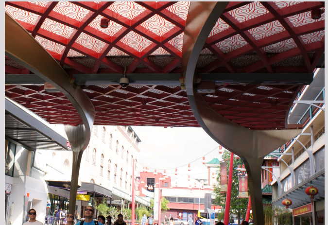
An example of public art integrated into building design
