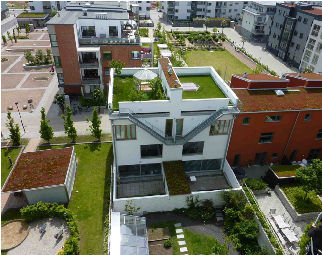
Careful consideration of the roof space with integration of services and greenery
