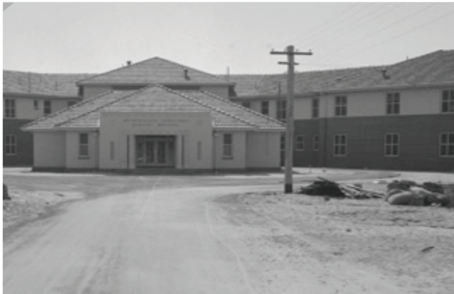
Archival Image 3 The new Infectious Diseases Hospital administration and ward buildings nearing completion in 1938 (Source: SLWA online image call no.09480PD)
