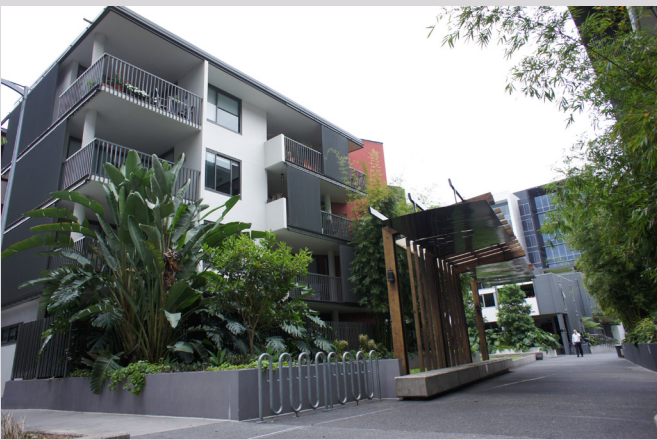
Corner residential ground floor apartment or terrace
