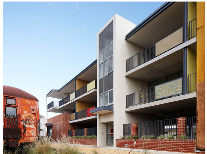
An example of a clearly defined pedestrian entry
