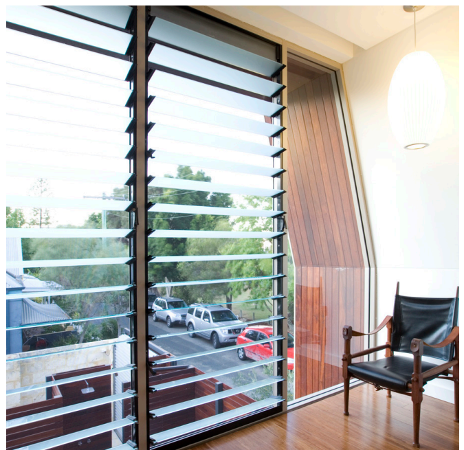
Surveillance: Maximise opportunities for casual surveillance from homes into the public realm whilst maintaining privacy of adjoining houses.
