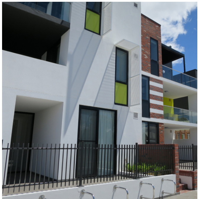
Fencing: An example of fencing that contributes positively to the quality of the area, promotes air flow and enables surveillance of the street (Blane Brackenridge Architects)
