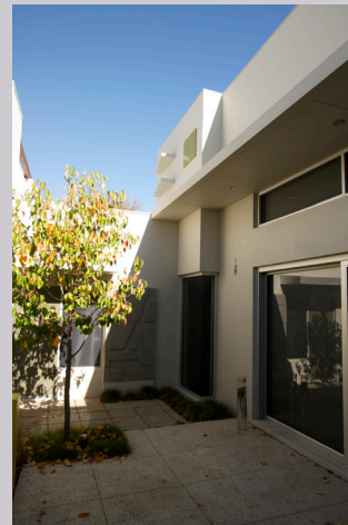
A combination of eaves and trees can provide shading to external paving and reduce the reflected heat load
