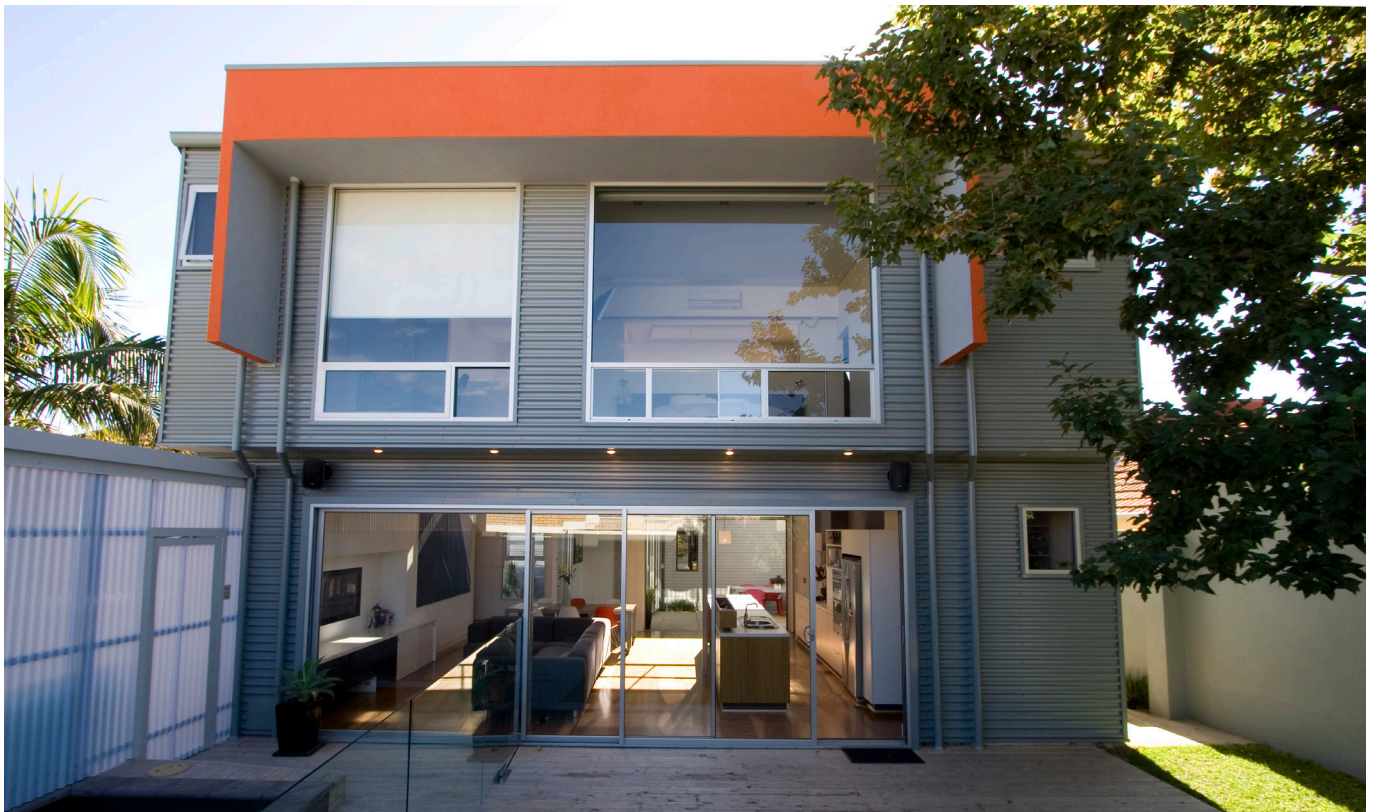
Solar Design: An example of an alternate eave solution to provide effective shading for openings and glazing
