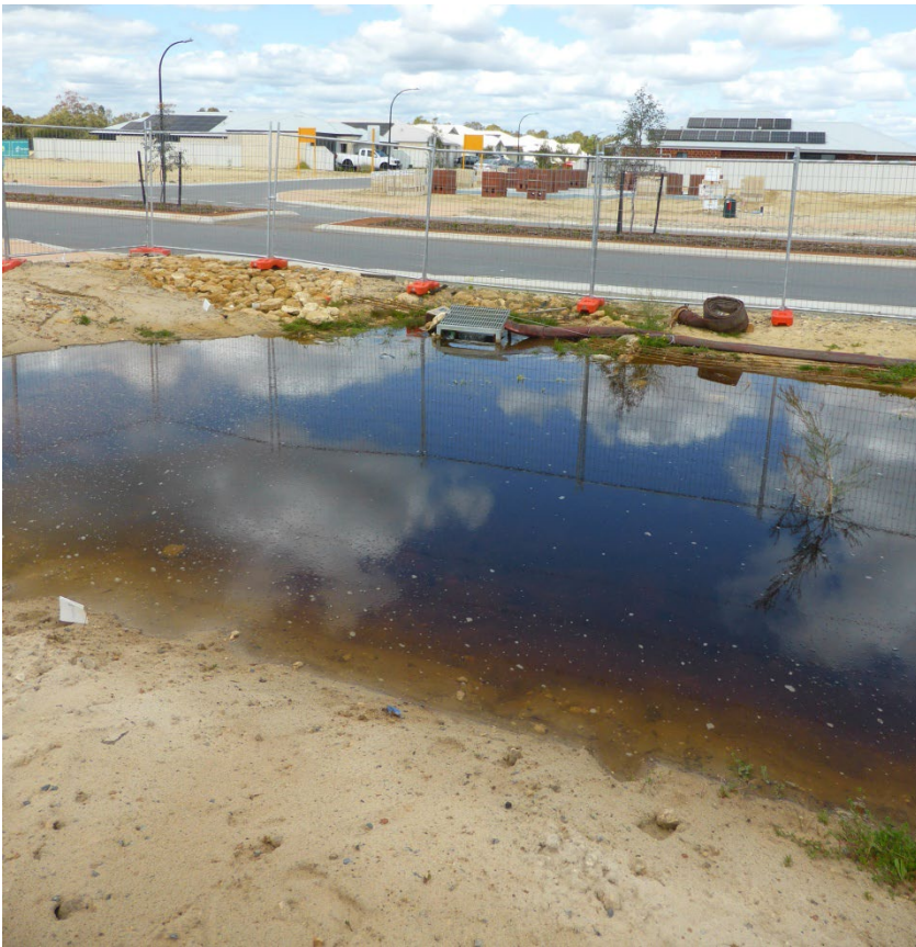
Drainage basins along Woollcott Ave, Brabham following rain event 27 th and 28 th September 29/09/24
