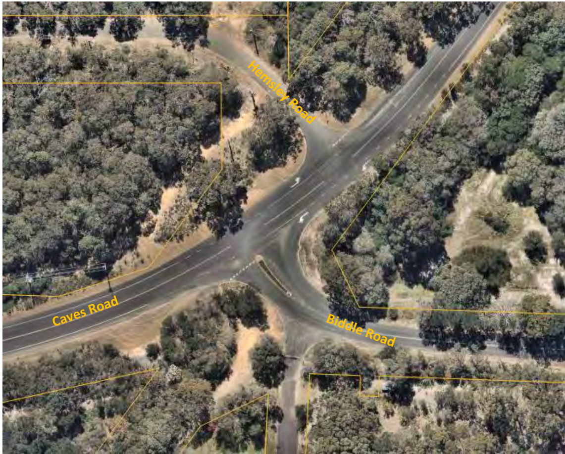
Figure 6-2: Biddle Road intersection with Caves Road
