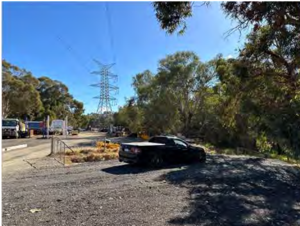
Photo 03: Power transmission lines
