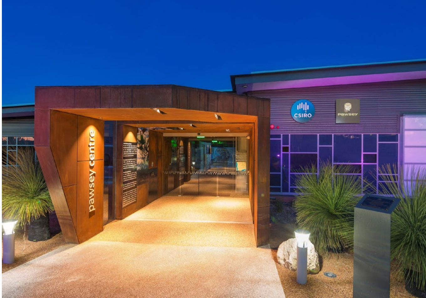
Pawsey Supercomputing Research Centre in Western Australia. CREDIT: Pawsey.
