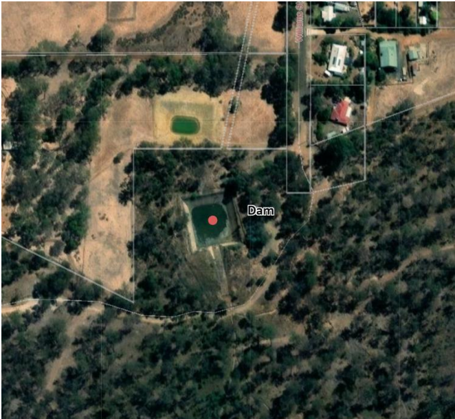
Aerial view of Railway Reserve dam
