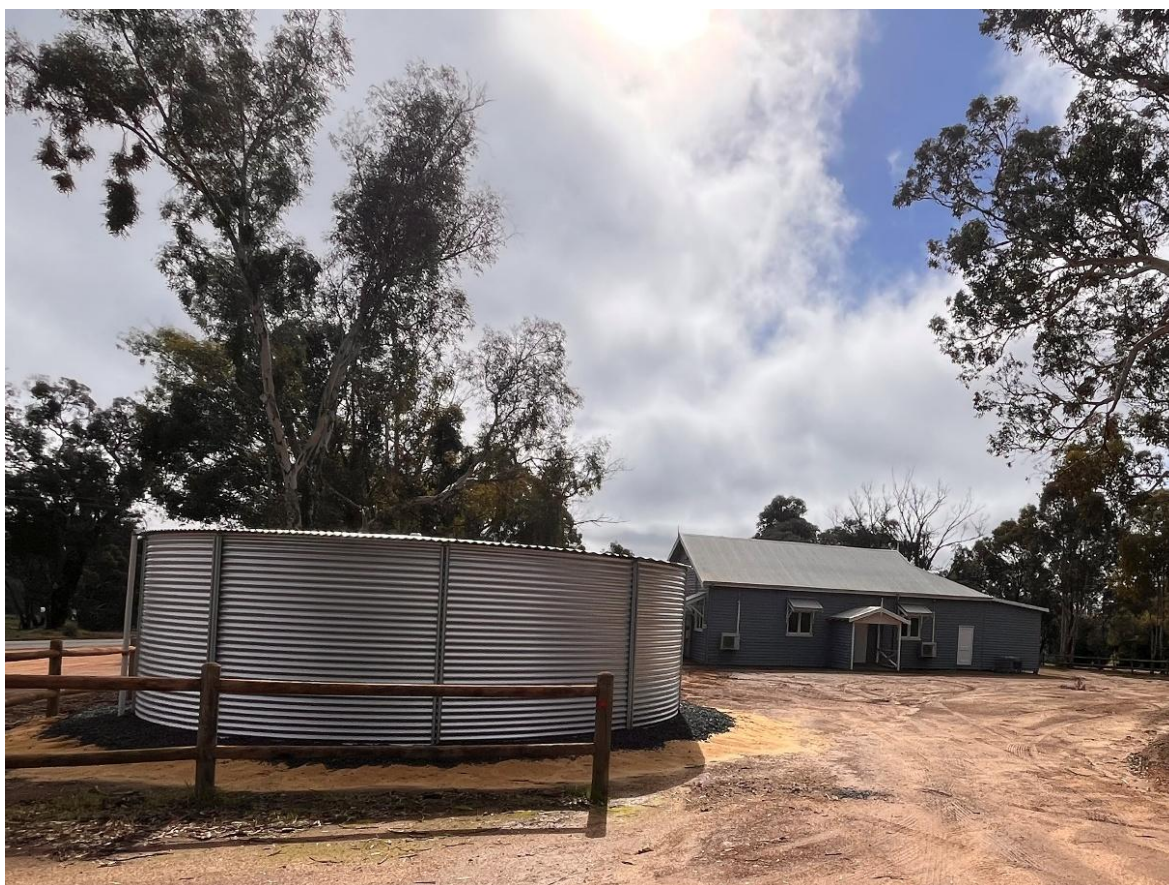
Mayanup Hall fire emergency tank
