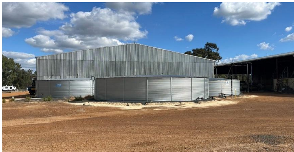
Three of the six tanks at the site
