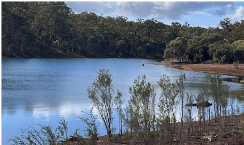
Reservoir Road dam
