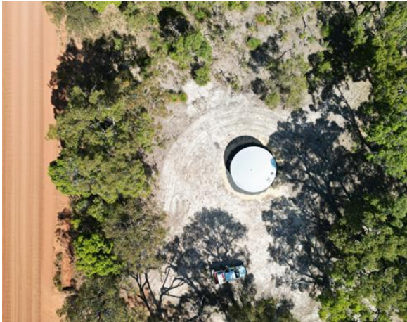
Aerial view of Tonebridge fire emergency tank
