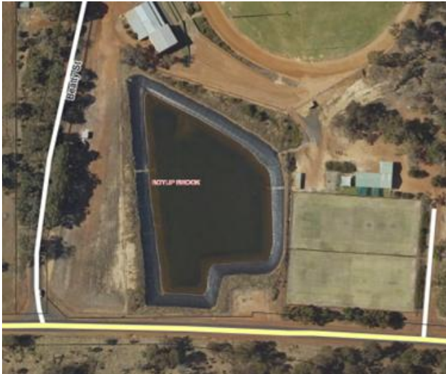
Aerial view of Sporting Rec dam
