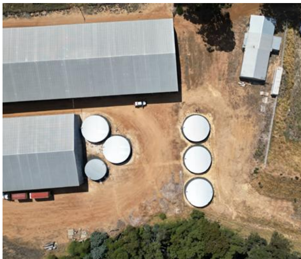
Aerial view of Flax Mill tanks
