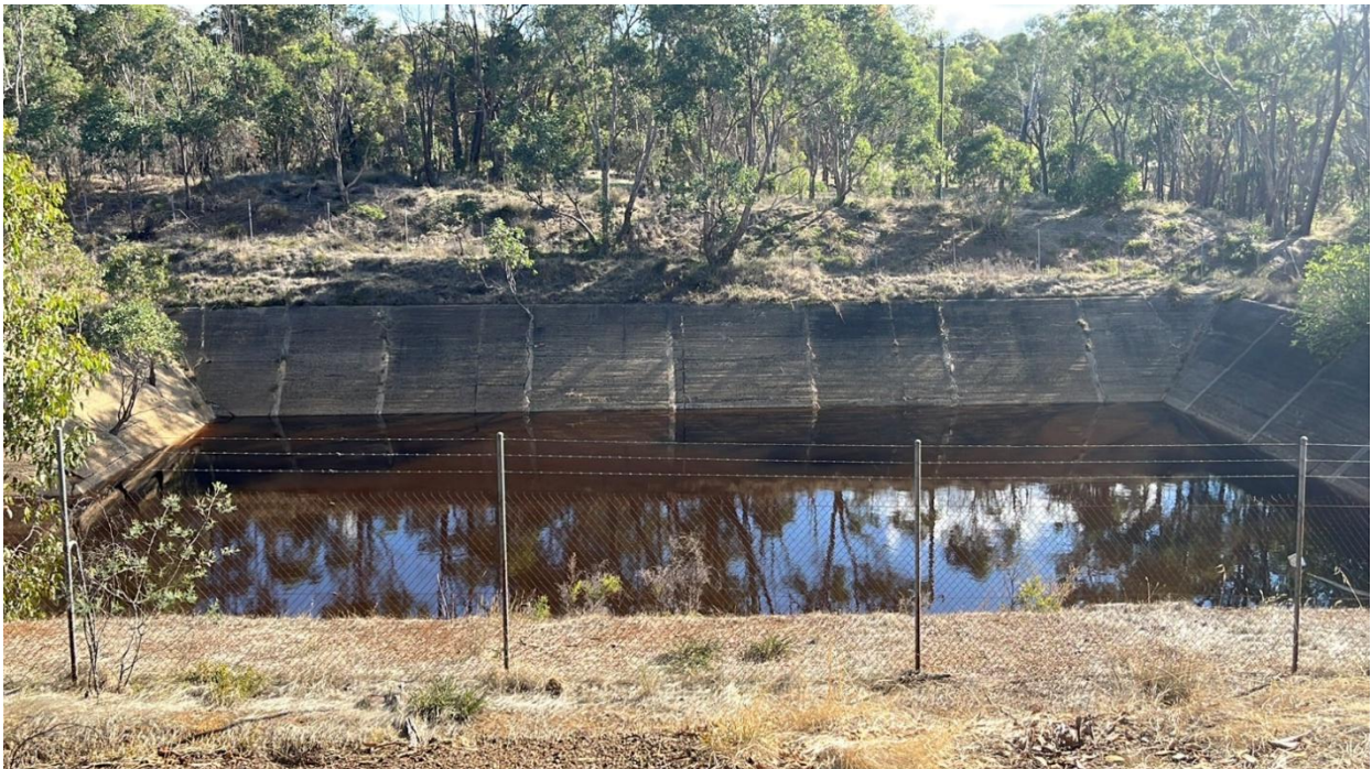
Railway Reserve dam
