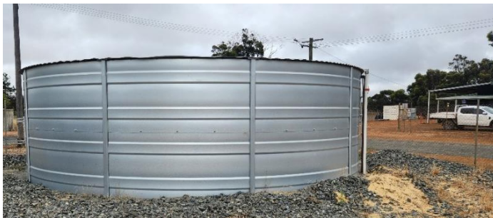
Tambellup Shire Depot tank 2
