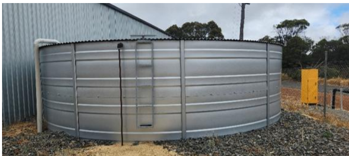
Tambellup Shire Depot tank 1
