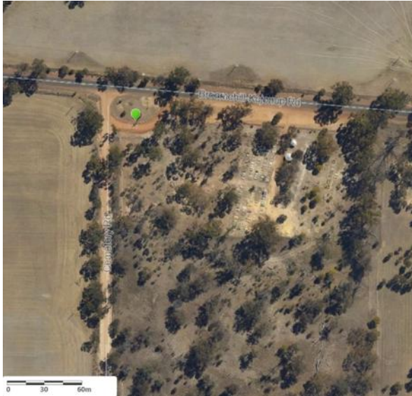
Aerial view of Cemetery standpipe
