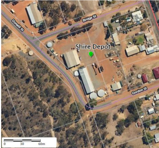
Aerial view of Tambellup Shire Depot
