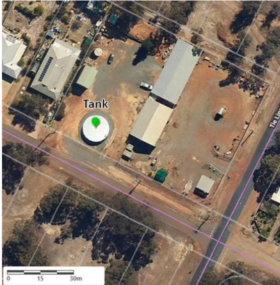
Aerial view of Broomehill Shire Depot
