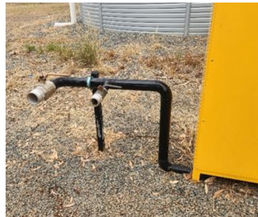
Swipe card outlets
