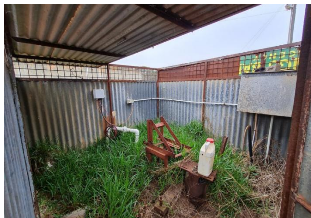
Inside pump/bore housing
