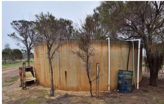
Anderson's Bore 2 tank
