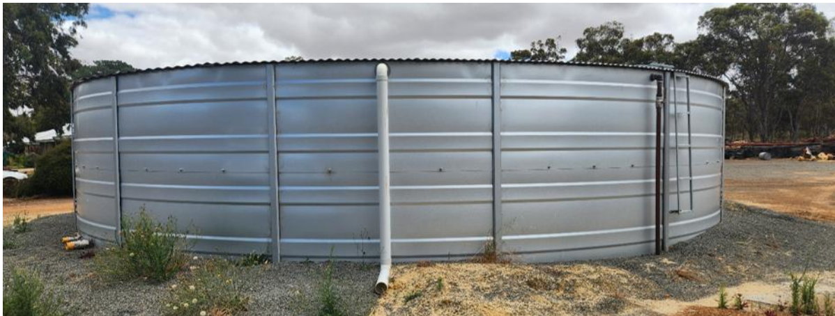
Broomehill Shire Depot tank
