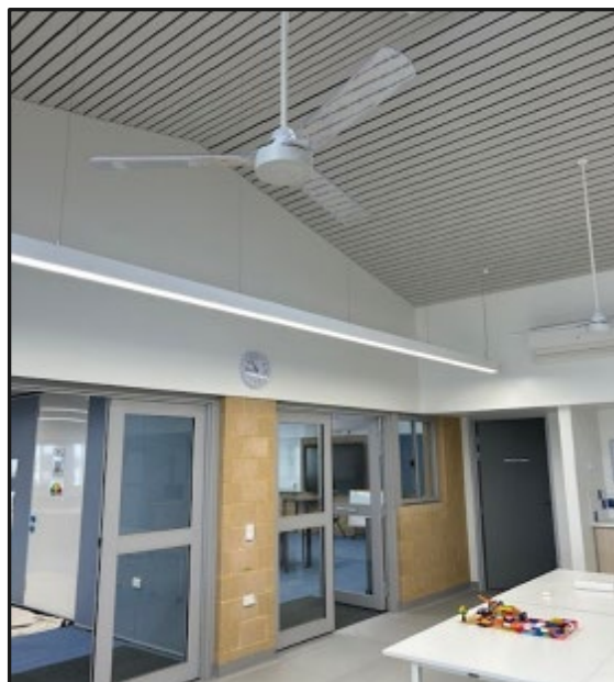
Figure 5.2 – Ceiling Fans Used in Learning Spaces
