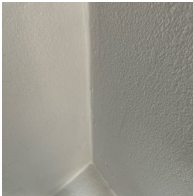
Figure 2: Well prepared junction in shower and correctly applied bond breaker fillet.
