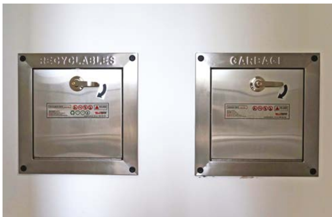
Photo 4.17a Dedicated recycling and waste disposal chutes allow source separation and recycling.
