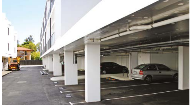
Photo 3.9b Tandem bays can provide increased spatial efficiency.
