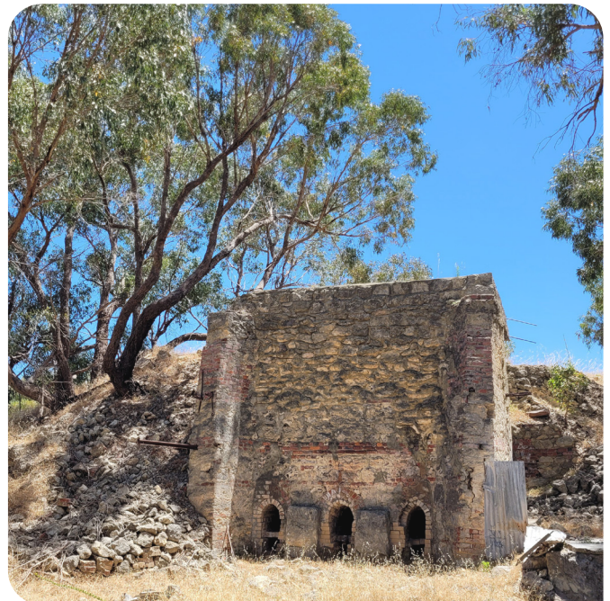
Above: The heritage-listed Spiers lime kilns are a distinctive local feature
